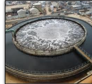
Activated Sludge Process (ASP)
